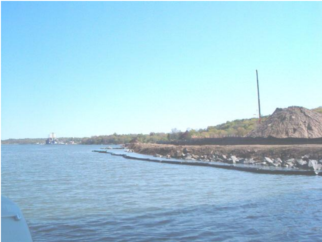
Construction of Bryant Landing development near CSHH #7 (Photo by Carol DiPaolo)
